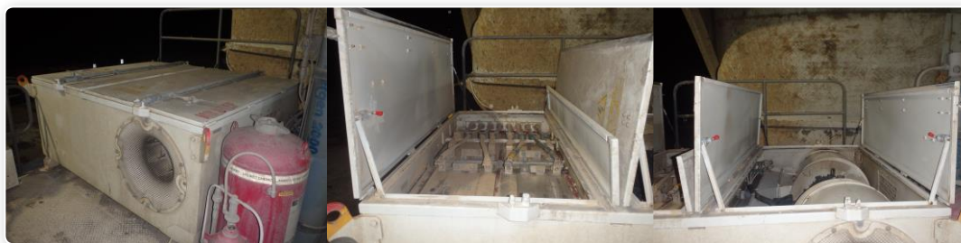
Modified Grid Box Covers and Opening Arrangement
