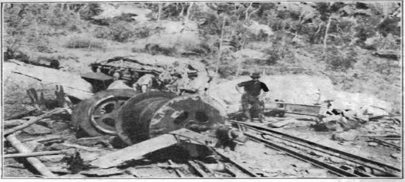
THE CABLE DRUMS, BLOWN 50 FT. FROM THEIR FOUNDATIONS.
