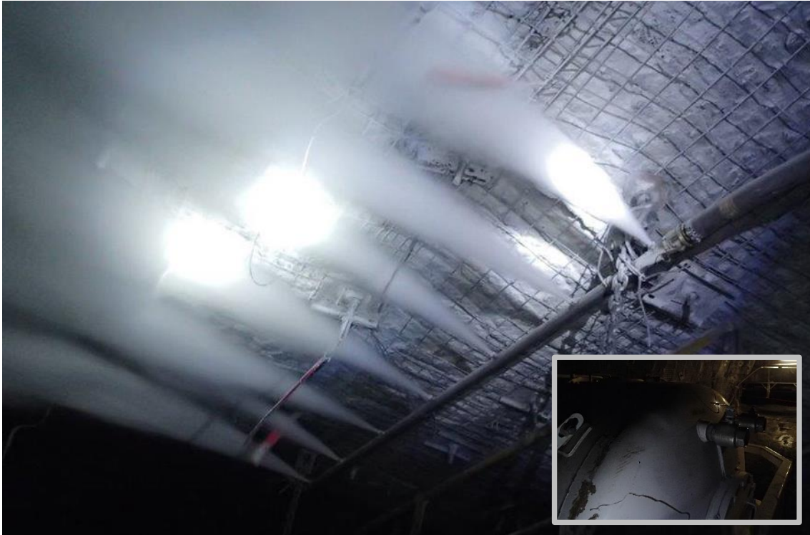
Pressurised Pod (Spray Bar) Method of Application
