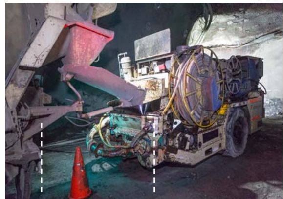
Picture 2 - Interaction Zone between Agitator and Shotcrete
