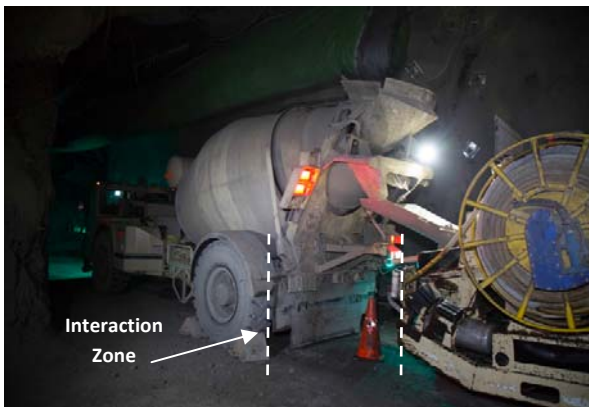
Picture 1 - Interaction Zone between Agitator and Shotcrete
