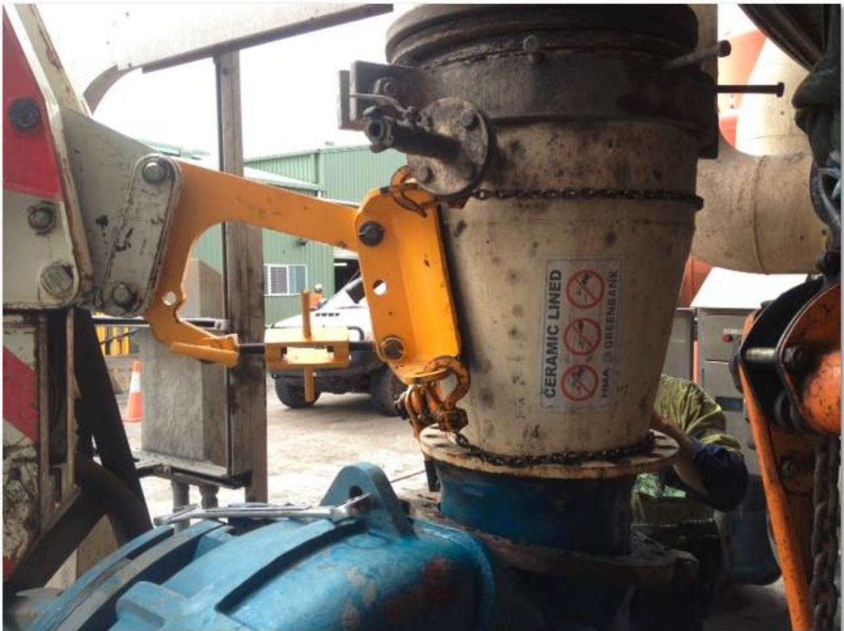
Fig.4 New Acland Coal's Multi-Fit Pipe Lifting Attachment shown in the process of installing the discharge spool from a Metso MM-400 Pump after the pump has been inspected & adjusted.
