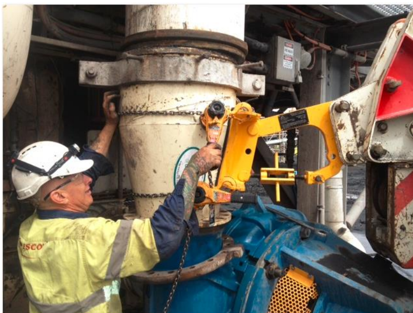
Fig.1 New Acland Coal's Multi-Fit Pipe Lifting Attachment shown in the process of being attached to the discharge spool from a Metso MM-400 Pump.
