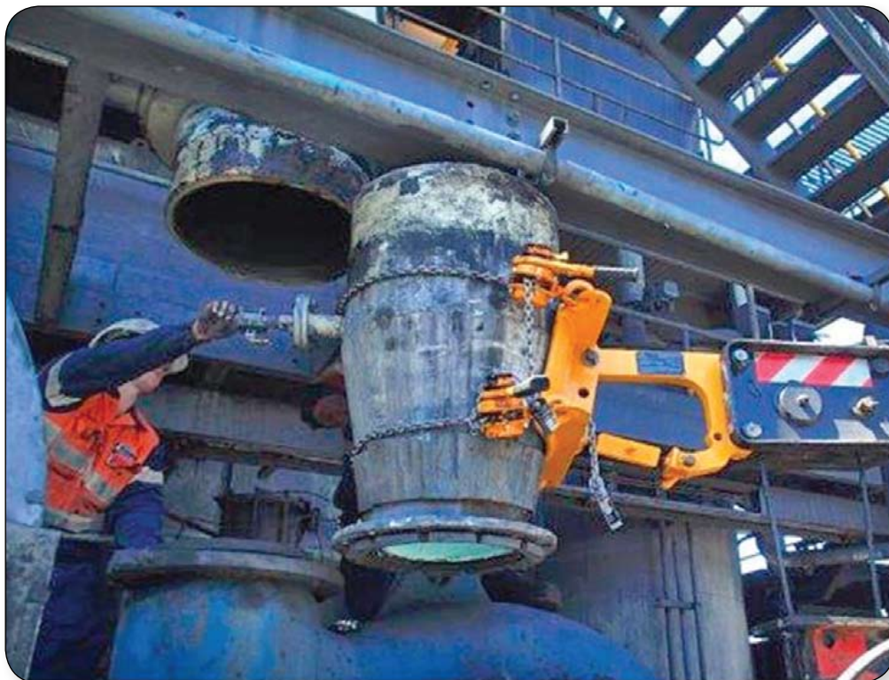
Fig.1 New Acland Coal's Multi-Fit Pipe Lifting Attachment shown in the process of removing a discharge spool from a XG-350 Metso Pump.
