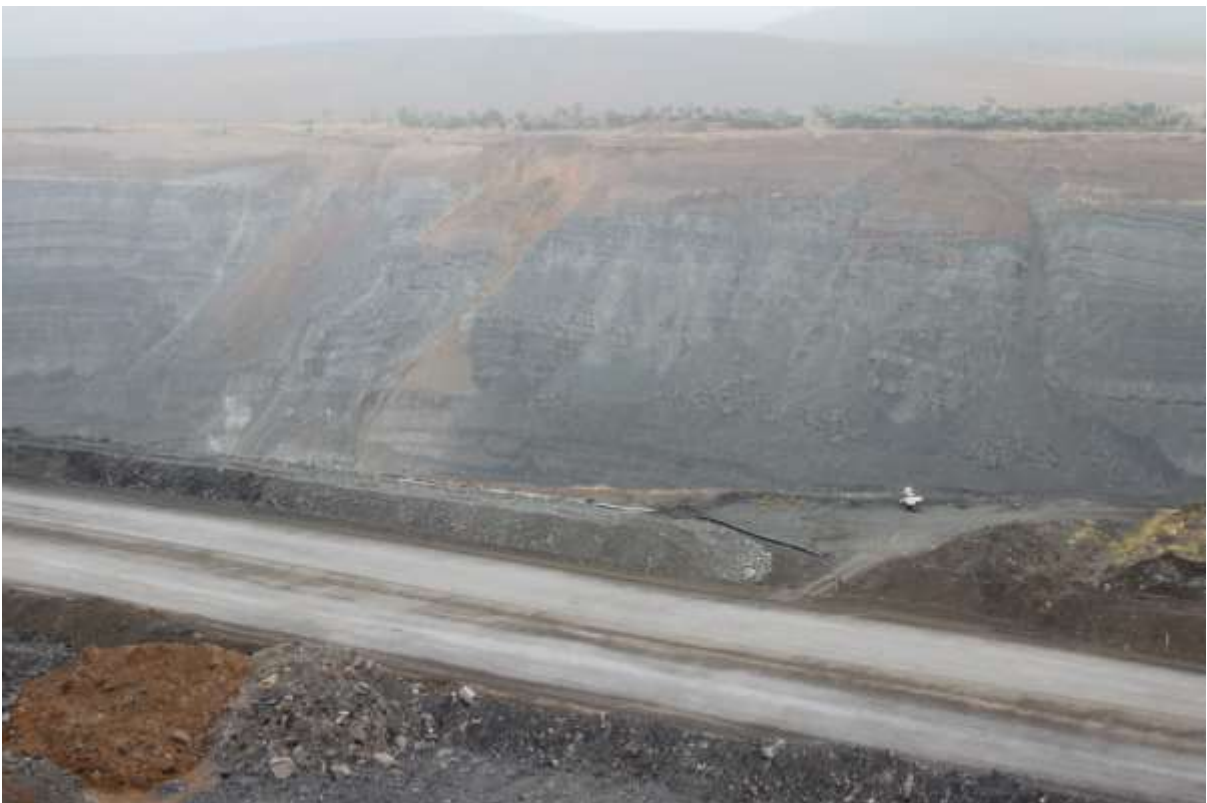
Figure 10 Photograph taken 14 June 2014 showing slope stability radar continuing to monitor highwall instability
