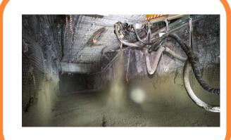
principles where applied to achieve an excellent outcome of being able to spray the floor at a thinner thickness than what we would traditionally using concrete dropped from boreholes to LHDs then transported to the area for dumping and spreading by equipment roughly and to a smother surface by
