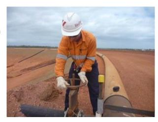
Figure 1 Manual method previously used to open and close valves
