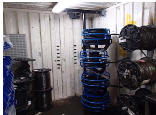
Picture 2. Hose reeler installed in container
