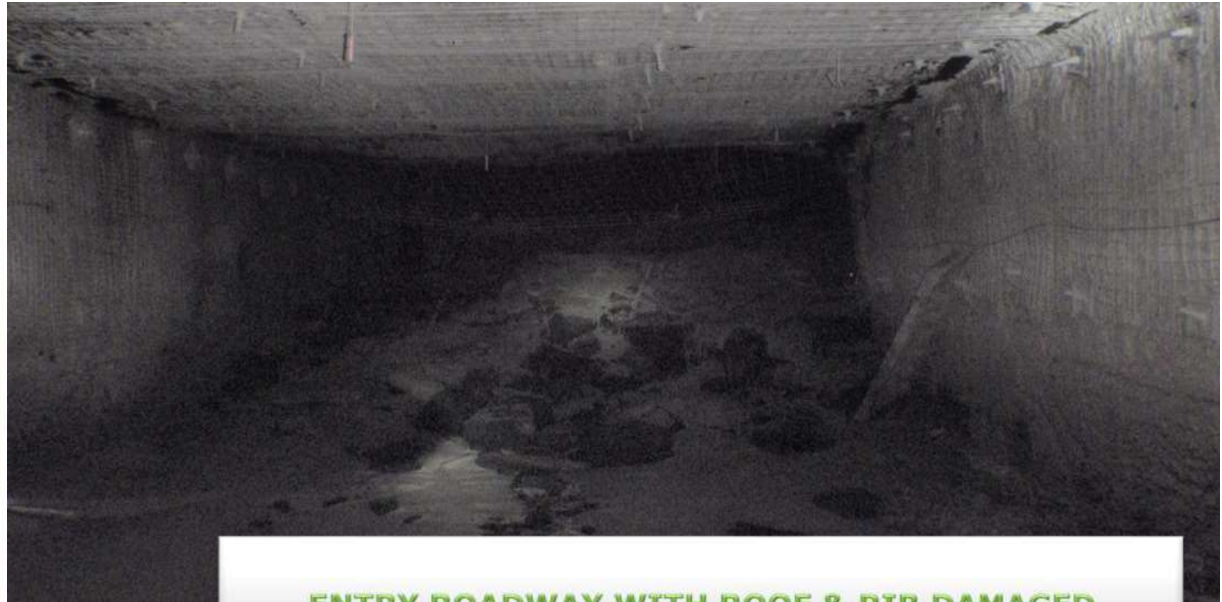
ENTRY ROADWAY WITH ROOF & RIB DAMAGED
