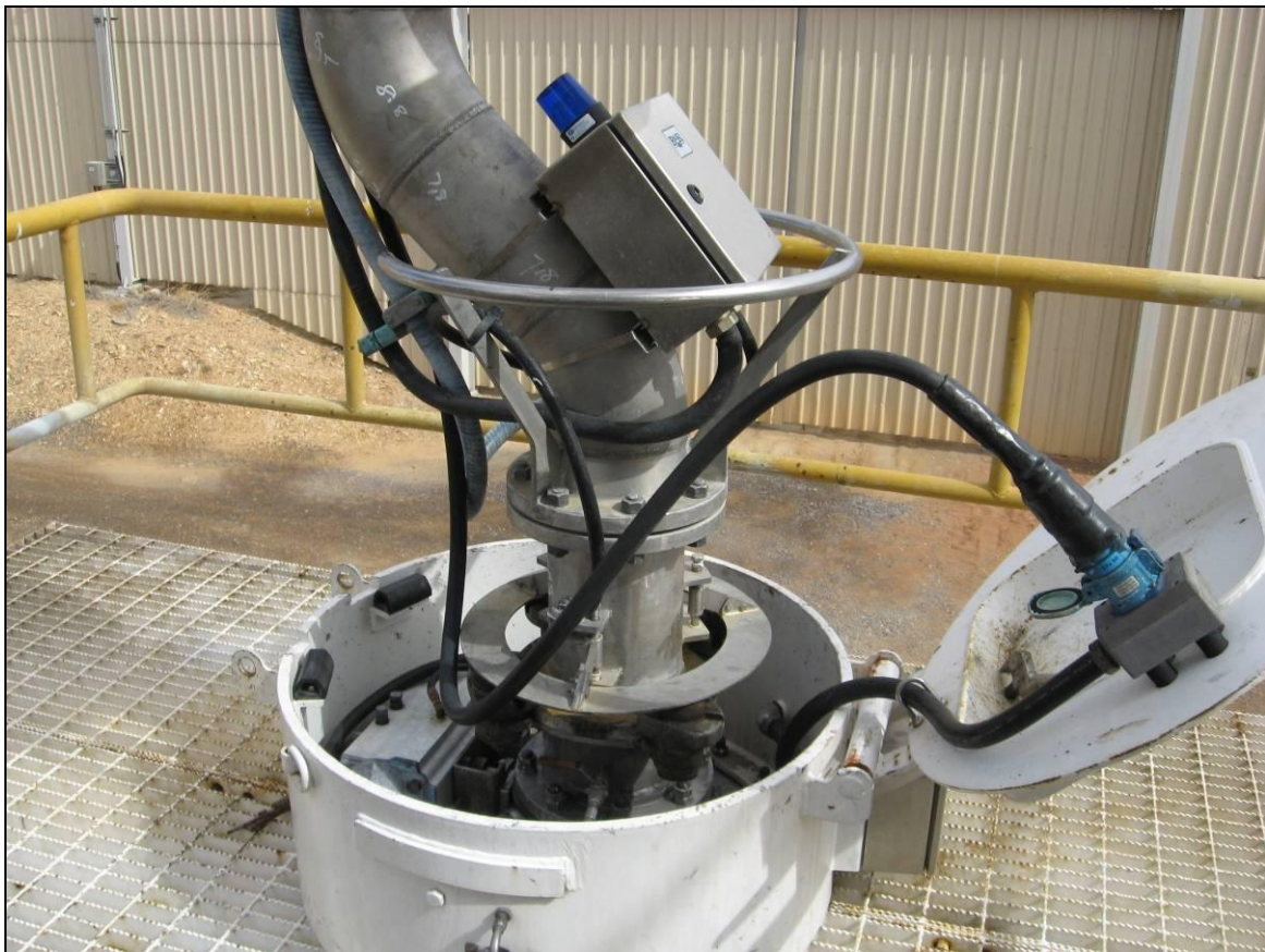
Acid Unloading Arm with Sensor system mounted directly on top.
