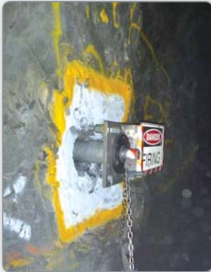
Photo 2: Telescopic Barricade installed but not grouted
