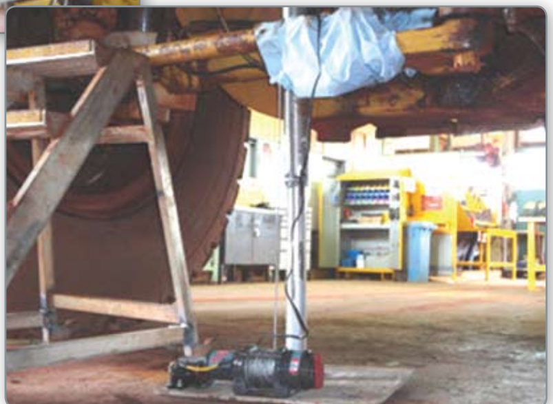
Figure 2: Jig extended into place
