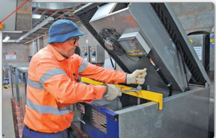
Figure 3: Lifting up drive shaft belt using tool
