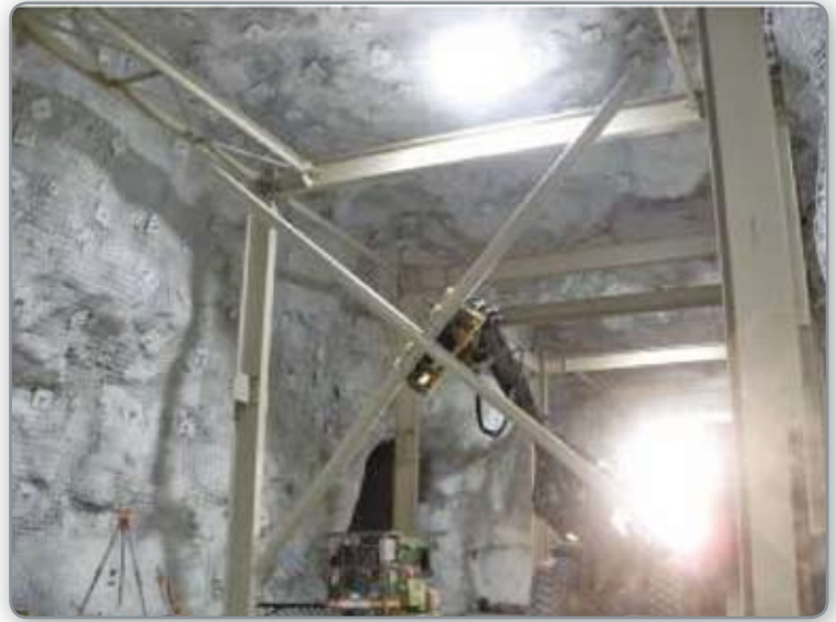
I-Beam installation on site
