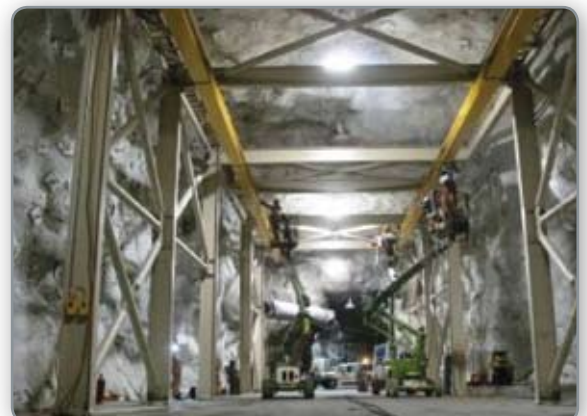
Underground workshop crane structure installation
