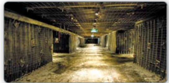
Roadway in Myne Start training complex
