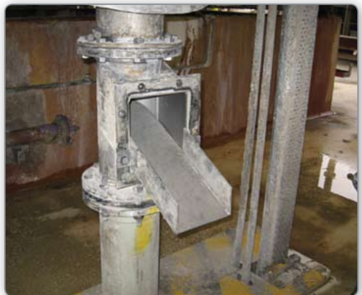
Scale Diverter Chute in place
