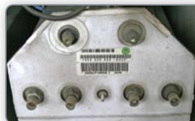
Image 4: New busbar produced by manufacturer with modified design.
