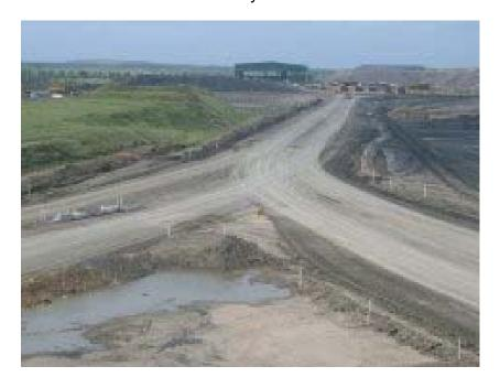
Y- intersections should be modified as shown below. A single intersection should be changed to a simple T-intersection at 90 degrees to the through road and a crossroad should be modified to a staggered T-intersection also bringing the side road to a 90 degree approach to the through road.
