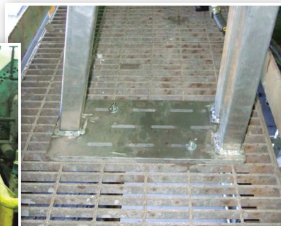
Photo 3 - Handrail Tester fixing to Johnsway mesh
