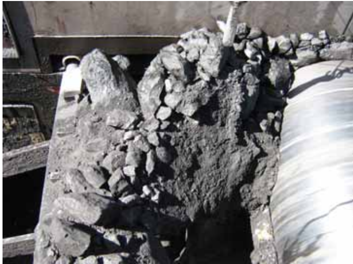
Figure 1: Large lumps of coal stuck in the head chute of the plant feed conveyor
