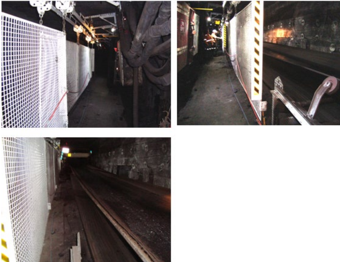
Figures 3 - 4 Underground set up
