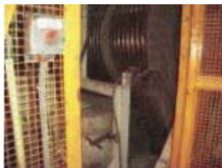
Rear of hoist drum area where operators accessed slack rope detector
