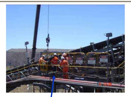
Lifting of the load was well controlled. The Supervisory Host ensured the area was clear as the load was descending Lifting area was barricaded and a spotter present
