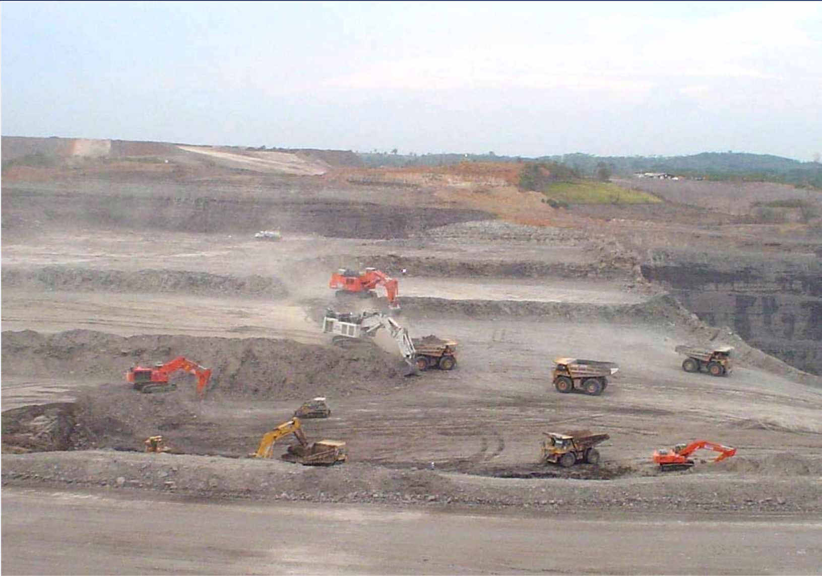
Excavator & Truck Fleet
