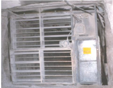
Figure 7 An example of a louvre regulator.
