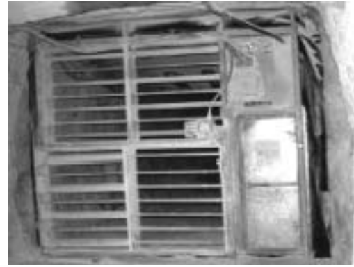
Figure 7: An example of a louvre regulator.
