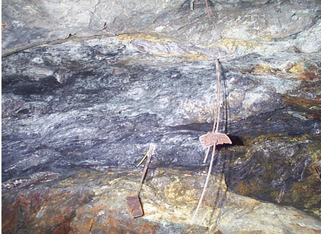
Figure 2: Unravelling of ground from around twin strand Garford cable bolts installed in the sidewall. Poor ground conditions associated with the J46 fault.
