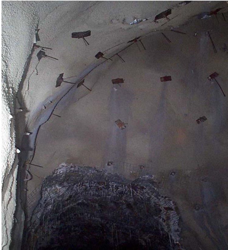
Figure 1: A 'cathedral' profile following rehabilitation.
