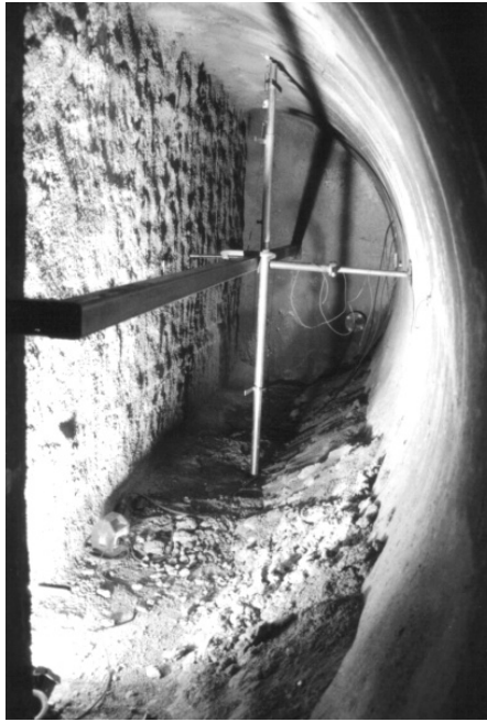
Figure 7. Internal view from the explosion side of the 325 mm thick Tcrete Seal. Note: the curvature of the Gallery shell (right) and the mounting for LVDT No 2.
