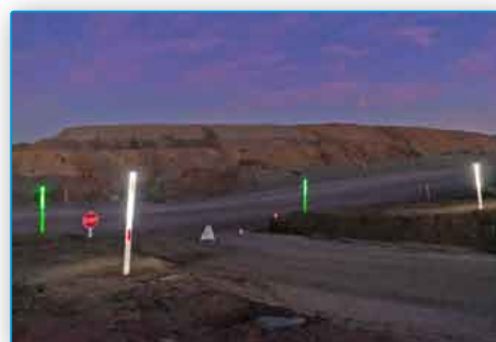
Fig3. Illuminated Guidance System- Road Crossing
