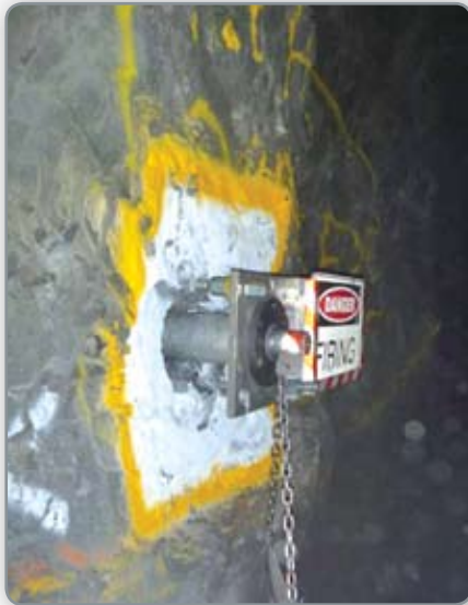
Photo 2: Telescopic Barricade installed but not grouted
