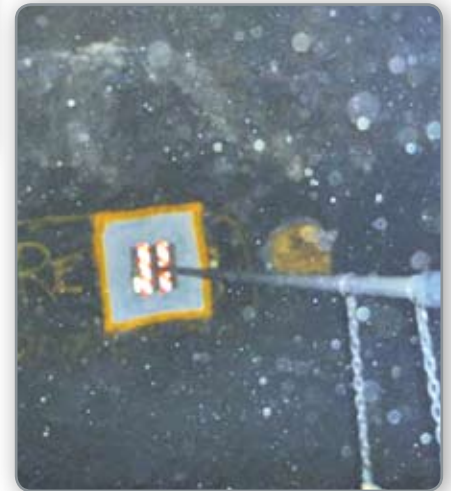
Photo 5: Telescopic Barricade locked into receiver on opposite sidewall
