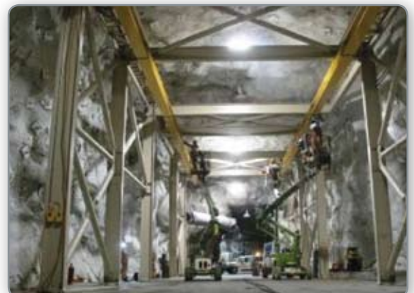
Underground workshop crane structure installation
