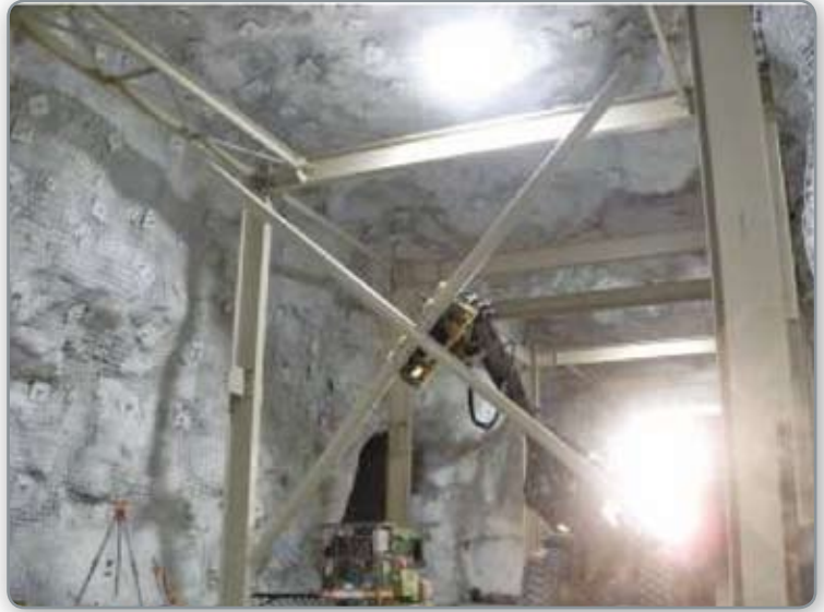
I-Beam installation on site
