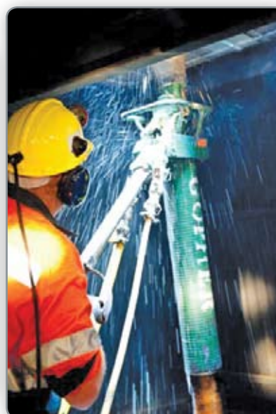
Trainee roof bolting in Myne Start training complex
