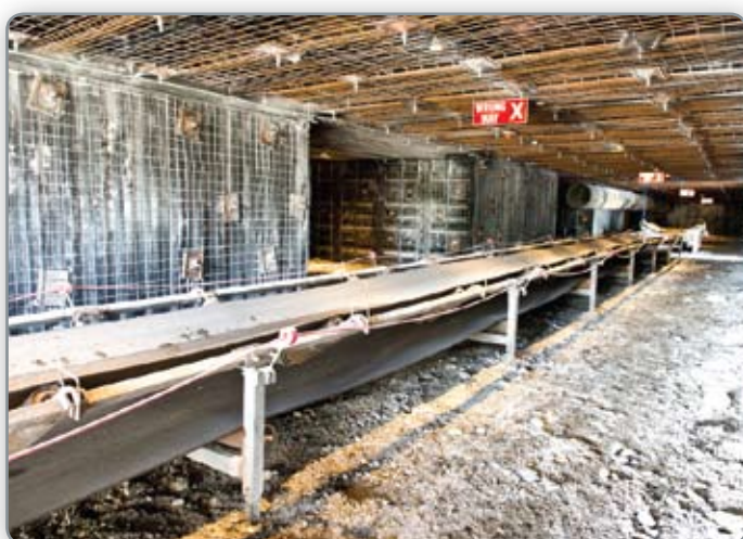
Working belt and roadway in Myne Start training complex
